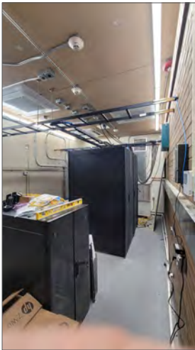
C. Campus server and Communications Room improvements at Administrative Center
